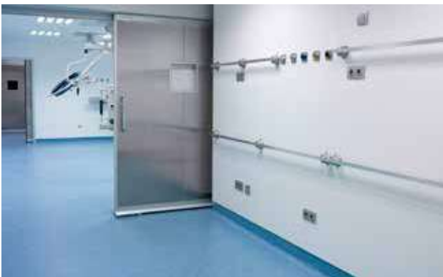
HOSPITAL PROVINCIAL (CASTELLÓN, SPAIN)
